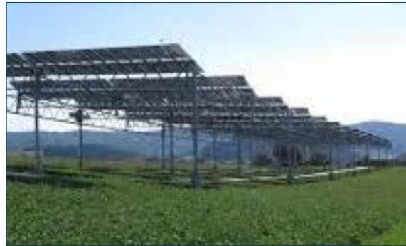
Different photovoltaics systems (BIPV, open field, Agro PV)
