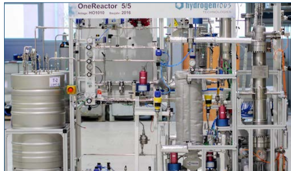
LOHC-One-Reactor (300 kW p )
