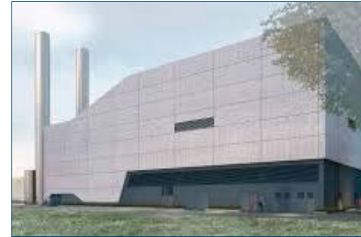
Combined heat and power plant (CHP) with H 2 co-firing
