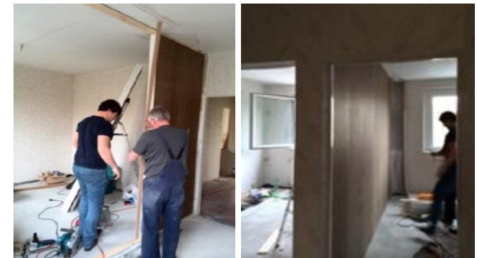
Test in concrete slab house, ready in 1h
