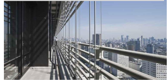
Sony City Osaka Building (shows TRL 9)
